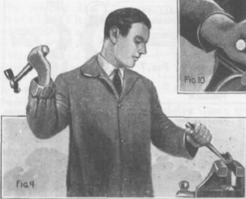
Left, End of Swing; Fig. 10, How the Chisel Is Grasped; Upper Right, Taking the Chip, and Lower Right, the Cape or Crosscut Chisel
