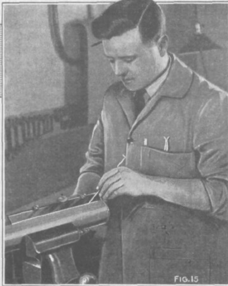
Fig. 14, Chipping a Broad Surface; Figs. 15 and 16, Laying Out and Cutting Keyseat on Shaft; Fig. 17. Holding Pulley for Keyseating and Fig. 18. Keyseat Square
