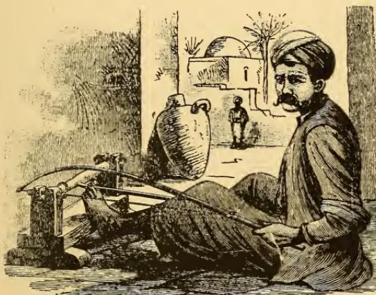
Fig. 2. Egyptian Lathe.
